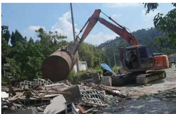
Fig. 2-16 Elimination of Outdated Production Factory
