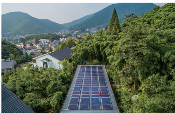
Fig. 2-14 Deqing Rural Rooftop Photovoltaic Installation
