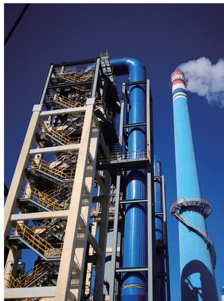
Fig. 2-28 Thermal Energy Saving Technical Transformation Project of Han Ye Company in Deqing
